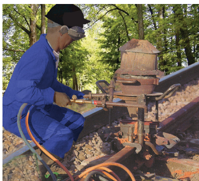
Figure 3.11 Thermit process for joining railway tracks
